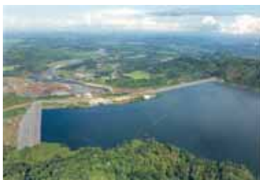
Bili-Bili Dam, the blue color of the water now turns brown due to sediment from Bawakaraeng Caldera wall collapse 45 km upstream.
