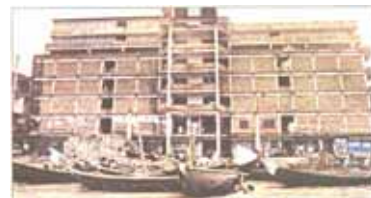
Photo 2 Encroachment near the Buriganga
